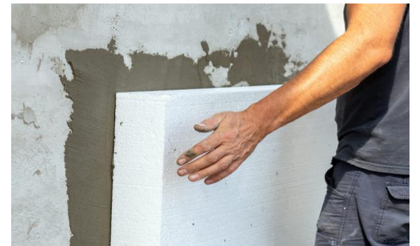
Complete External Thermal Insulation Systems (ETICS)
